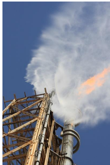
Picture: Hydroshield in operation.
