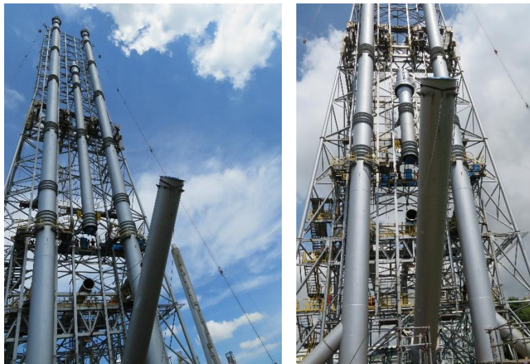
Photo: Lowering one of the sections of the riser of GSP6
