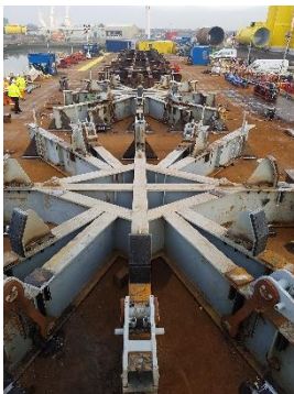
Picture: Barge with type 2 grillage
