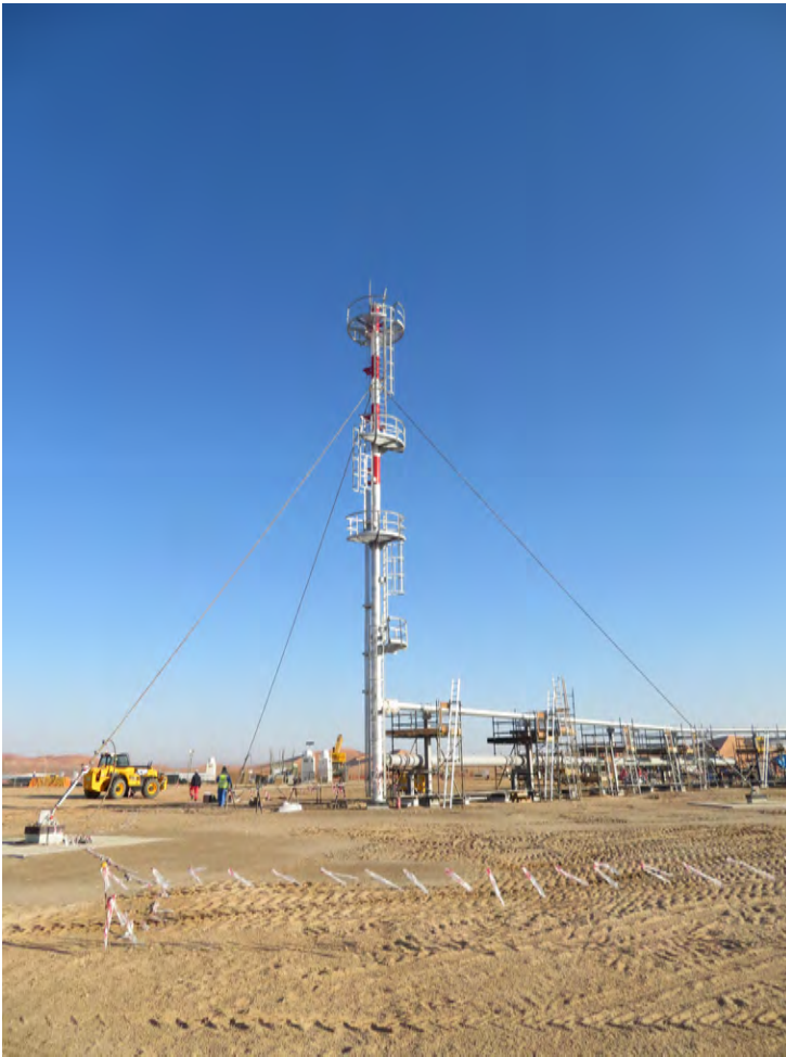
Photo: Guy wires tensioned according specifications
