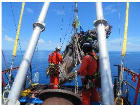
Picture: A frame and flare tip handling
