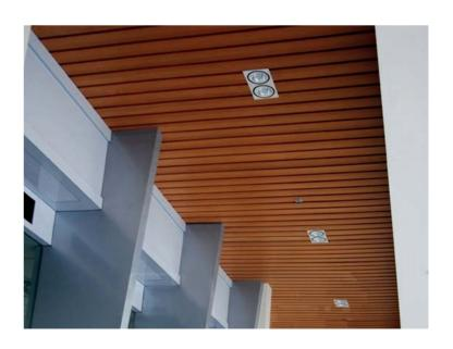
WARNING: any lights and other recessed elements must be fixed to a support structure and not directly on the plank.
