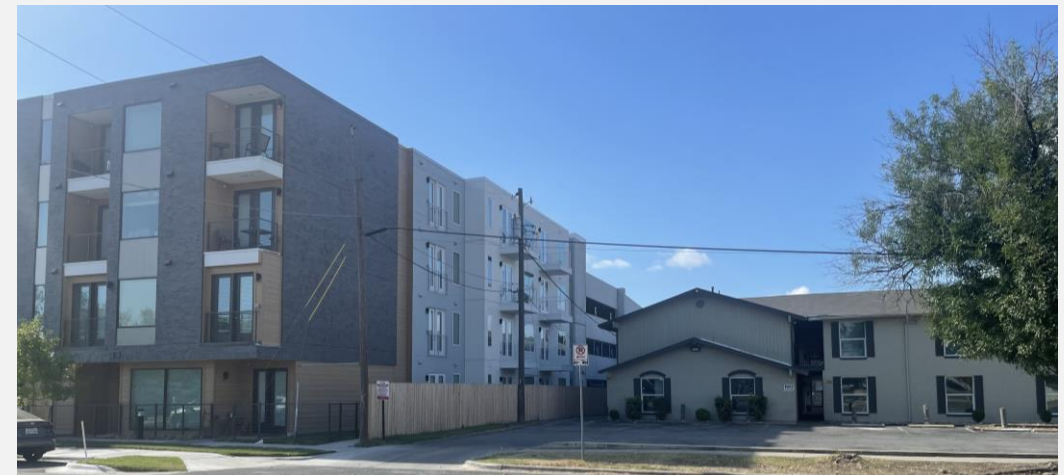
Neighboring properties in the same submarket that are clearly very different in age, price and amenities, and cater to different tenant bases,
