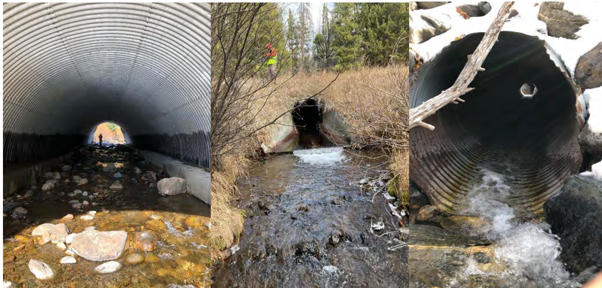
Figure 42 Aquatic Passage Assessment: Images of a “Green” Crossing (left), a “Gray” Crossing (middle), and a “Red” Crossing (right)
