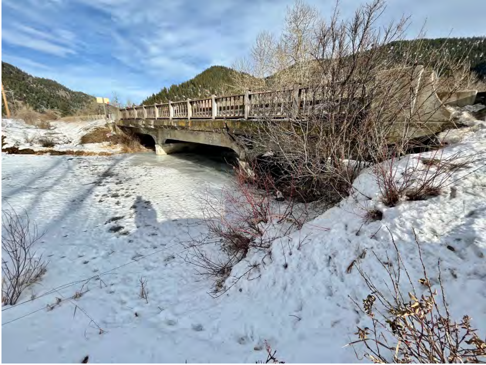
Figure 28 Spanish Creek Bridge (RM 68.1)
