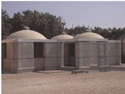
Figure 3. Load-bearing stabilized rammed earth building.
