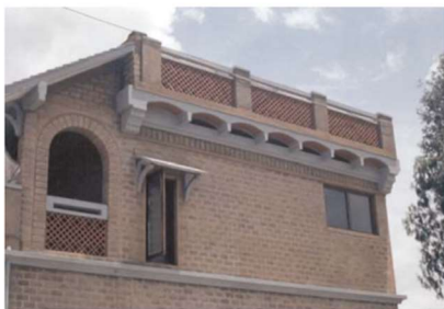
Figure 4. Composite masonry jack-arch roof system.
