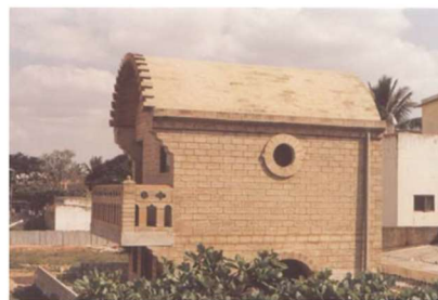
Figure 6. Unreinforced SMB masonry vault roof.
