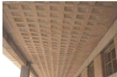
Figure 5. Ceiling of an SMB filler slab floor.
