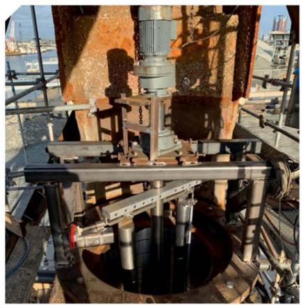
The new rudder stock was delivered with 4mm oversize and the pintle with 10mm oversize on the cones. The reason for this was to have sufficient material to machine in the rudder blade cones and be able to adjust the rudder blade cones if any misalignments were measured.
