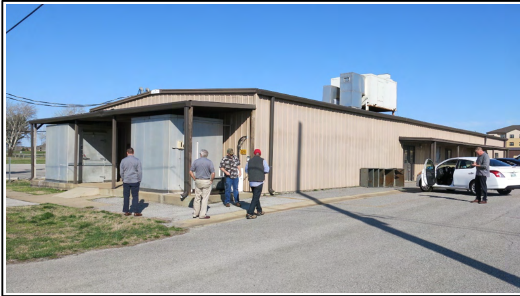
Figure 3. Exterior of Bldg. 2261—dining facility.
