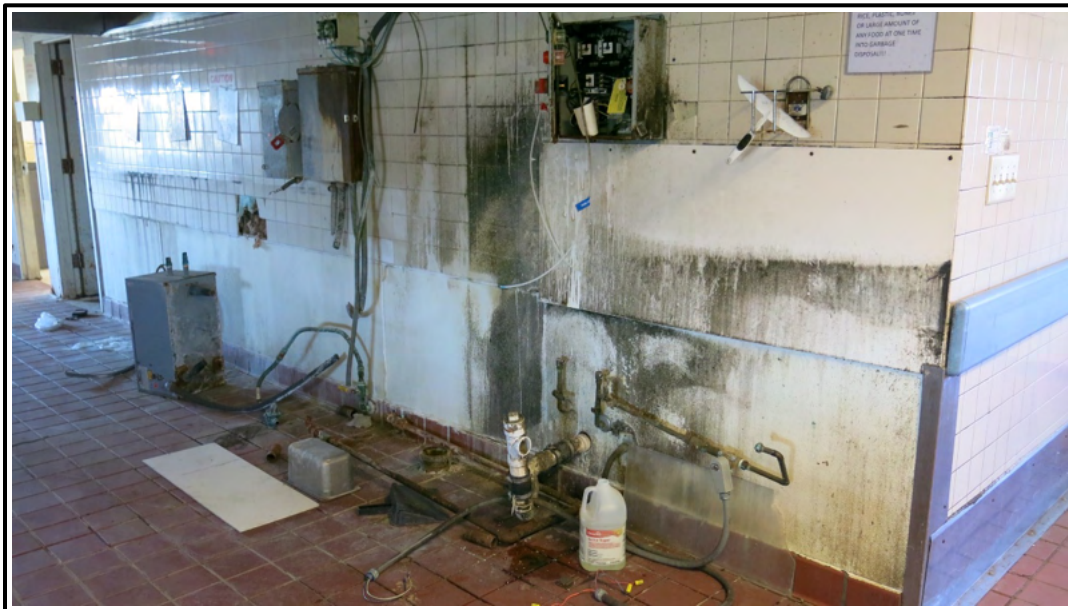
Figure 4. Kitchen area inside Bldg. 2261.
