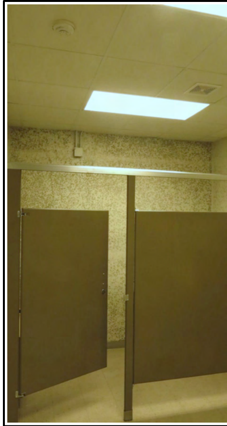
Figure 8. Bathroom area inside Bldg. 6733.
