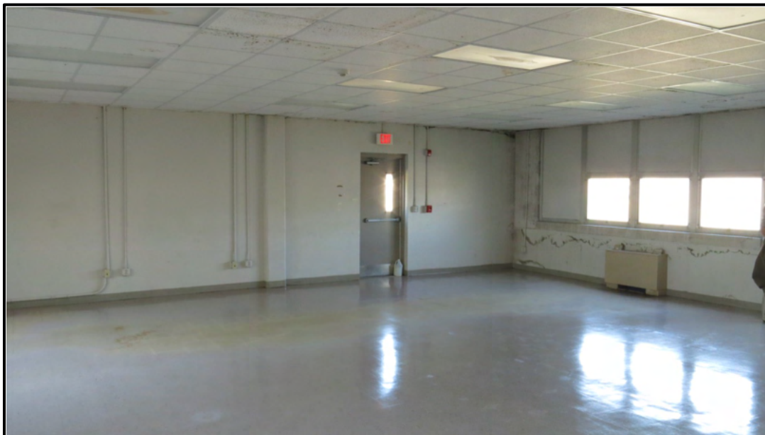
Figure 7. Classroom area inside Bldg. 6733.
