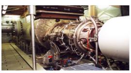
This installation is for an in-line gas compressor station utilised for land based gas transmission system where intermittent stations are positioned along the pipe route to build up pressure gas in the pipeline supported by line looping for the additional holding capacity.
