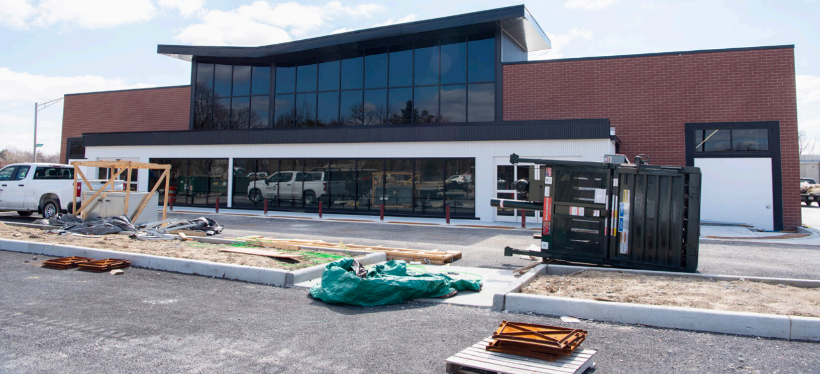
▲ The nearly completed Indy Fresh Market building.
