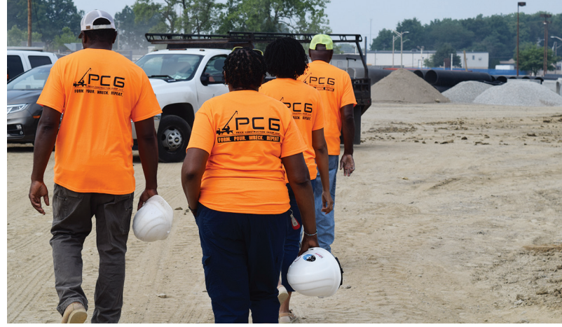
▲ Members of the Price family leave the 38th & Sheridan Project worksite to head back to the Price Construction Group, LLC office.
