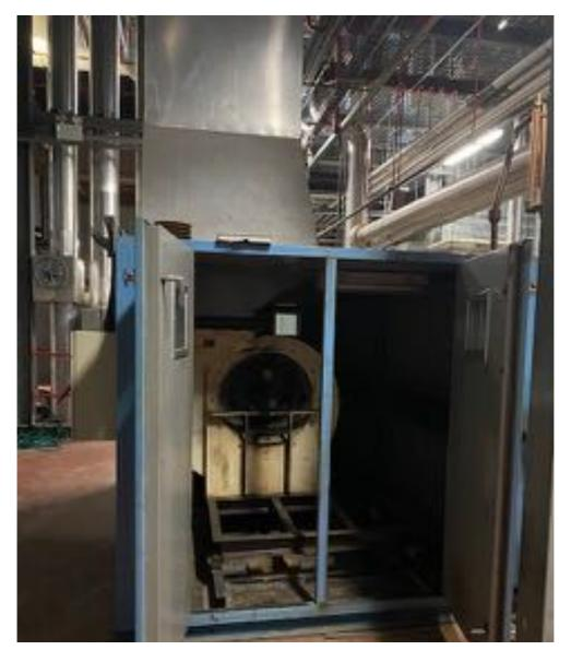
The installation of the 40 Package PHI units is a relatively simple process. Each unit has magnetic feet and can be attached to the inside walls of the AHU at the supply / main duct branch junction. Power supply is via a transformer and an isolated fused spur taken from the lighting circuit inside the AHU.
