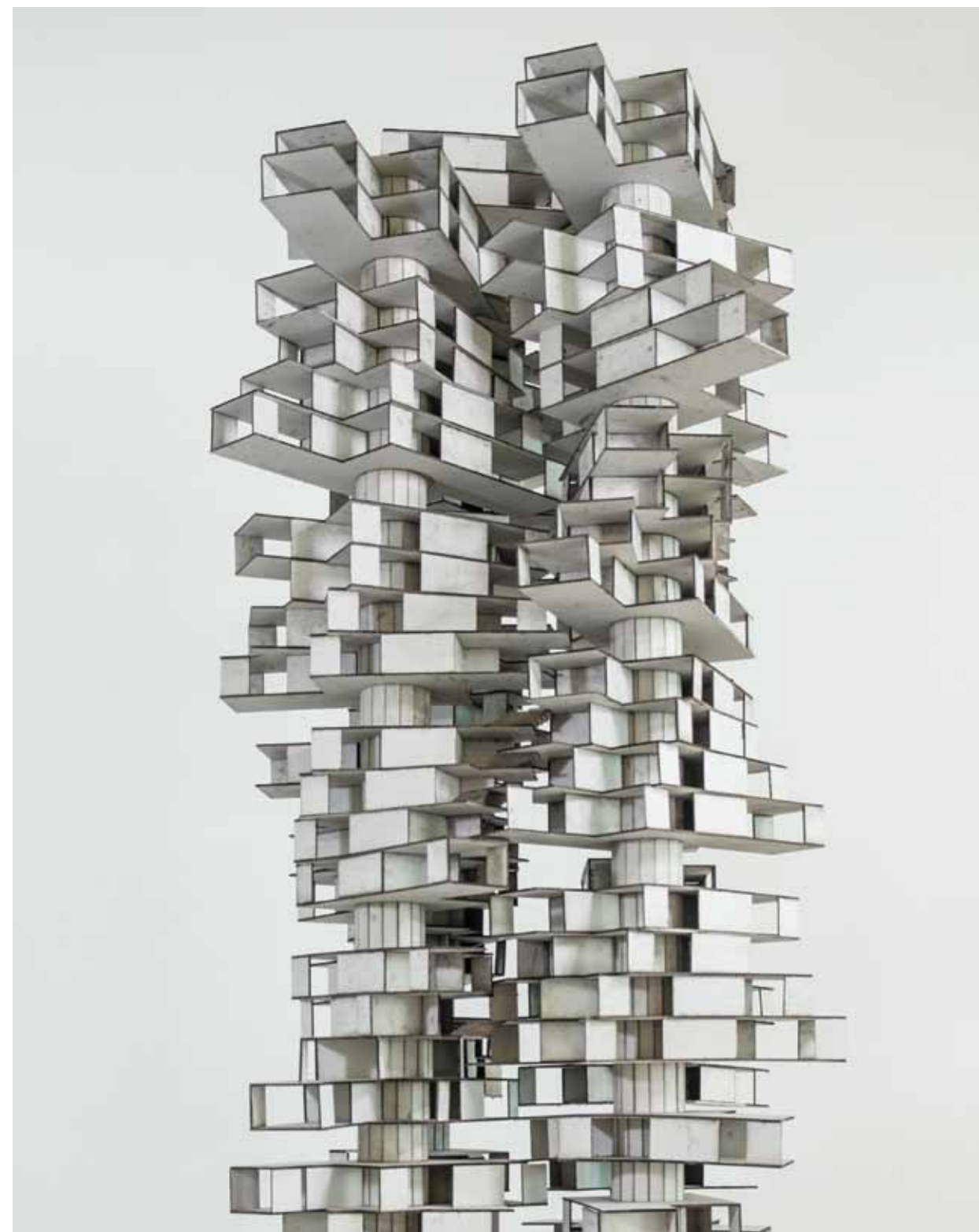
Tower 2 In the second tower the void decks are introduced. Every sixth floor is left empty, articulating clusters of residential units. These clusters act as Vierendeel trusses, leaving the void decks free of structure. The apartments rotate freely around their centre, creating different views and trying to connect to the next void deck cluster.
