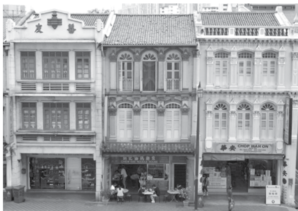
Shop houses represent the oldest urban typology in Singapore, containing shops, restaurants or cafes on their ground floor with residential unit on top
