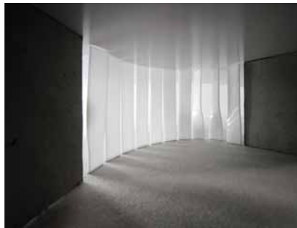
The deformed acrylic elements become the enclosing system and are placed in between the primary tectonic structure
