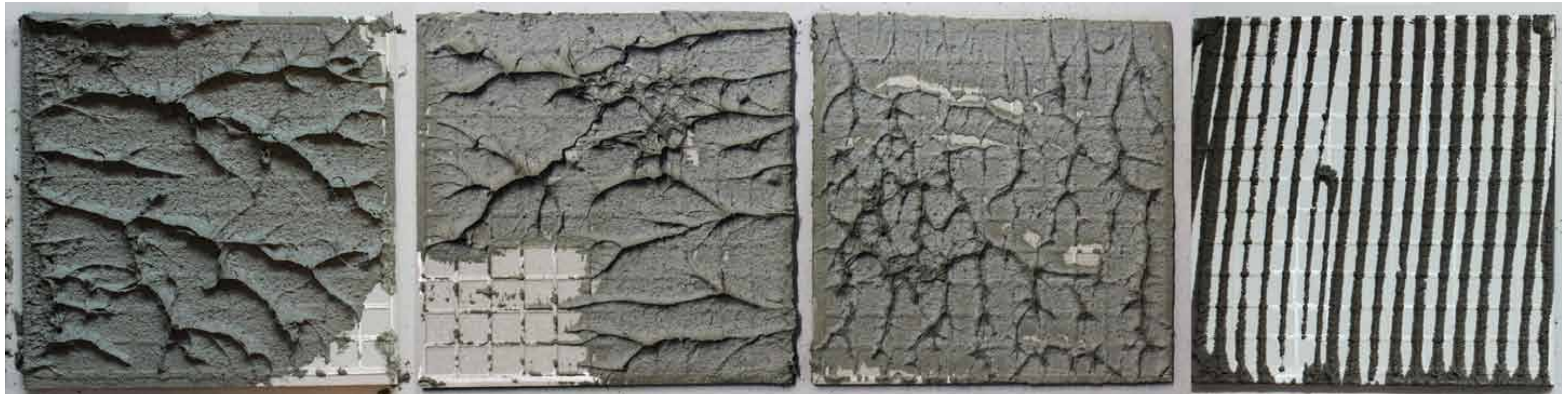
Fig. 13 Various states of the adhesive coverage of tile underside: (from left to right) special bedding movements + vibration, special bedding movements + vibration on an uneven adhesive bed, special bedding movements + vibration on a thinner adhesive bed, no special movements
