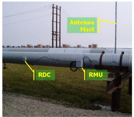
Figure 5 - Typical deployment
