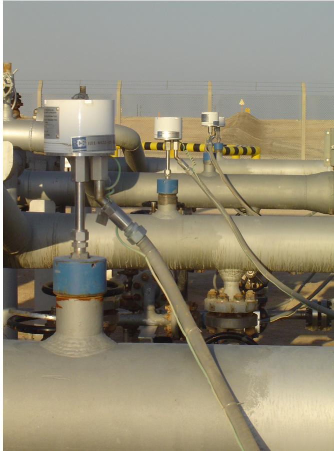
Figure 8 – Direct Coupling of Transmitter and Sensor
