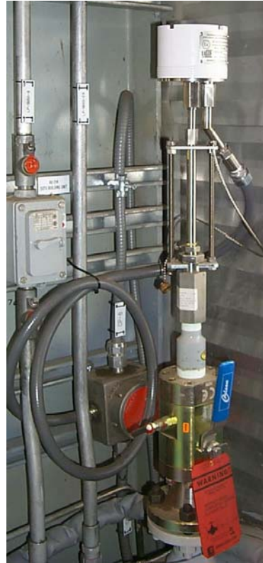
Figure 3 High pressure retrievable upstream probe and transmitter, and medium pressure process plant probe and transmitter
