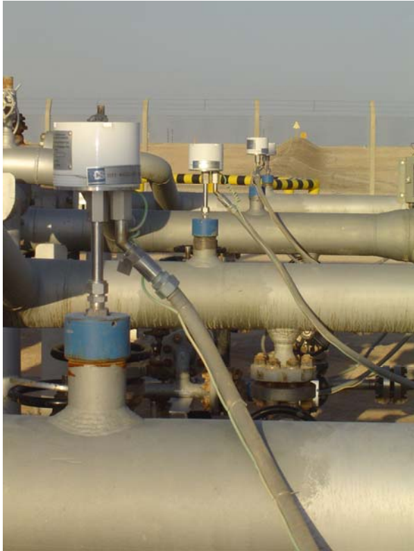
Figure 3 High pressure retrievable upstream probe and transmitter, and medium pressure process plant probe and transmitter
