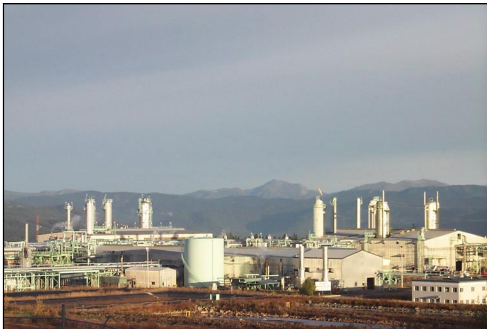
Figure 7 Pine River Gas Plant
