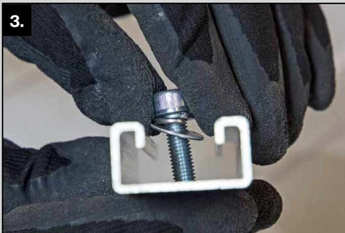
3. Assemble the 8 mm bolt, lock washer and washer and put through the pre-drilled hole in the mounting track.
