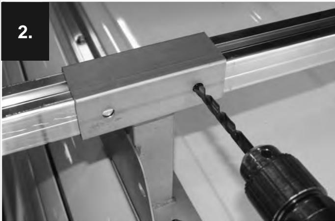
2. Using the predrilled holes in the mounts as guide, drill 5/16" holes through the crossbars.
