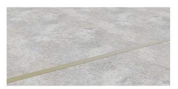
10. After the new slab/screed has hardened sufficiently, the top strips or extenders can be removed for re-use, simply pop/lift off using a screwdriver at one end to break the seal and free the strips - or alternatively leave in situ, if required.
