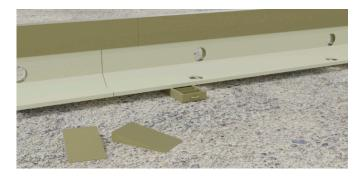
3. If extra height is required, place a pair of wedges under the rail base, close to where the pins are to be driven through, adjust to height required.
