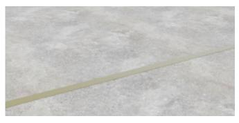
8. After the new slab/screed has hardened sufficiently, the top strips or extenders can be removed for re-use, simply pop/lift off using a screwdriver at one end to break the seal and free the strips, or alternatively leave in situ if required.
