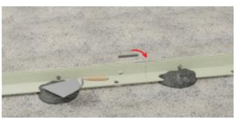
5. Trowel over excess concrete/mortar onto rail base, and bench up the sides, ensuring correct alignment and height of rails, especially at joints. straight coupler alignment ferrules are available if required –simply pop into the top slot on the rails where they join – allow concrete/mortar to cure.
