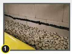
Apply Stego Mastic to the foundation wall at the anticipated edge of the subsequently applied Stego Wrap at the height of the slab or impediments.
