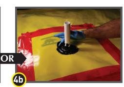
Seal around the base of the pipe with Stego Mastic. Note: apply using disposable glove, paint brush, or similar.
