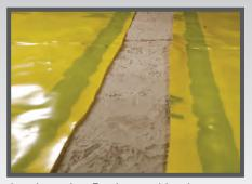
At a Location Designated by the Design Team: Seal Stego Wrap to concrete with Stego Mastic.
