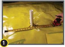
Cut a detail patch to a size and shape that creates a 150 mm (6") overlap on all edges around the void space at the base of the pipe.
