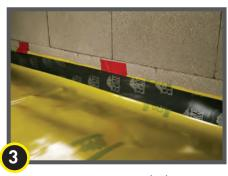
Apply the entire 75 mm (3") width of Stego Crete Claw Tape on the perimeter edge of Stego Wrap.
