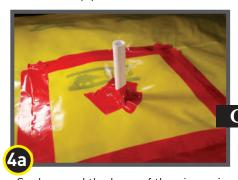
Seal around the base of the pipe using Stego Tape. **OR...**
