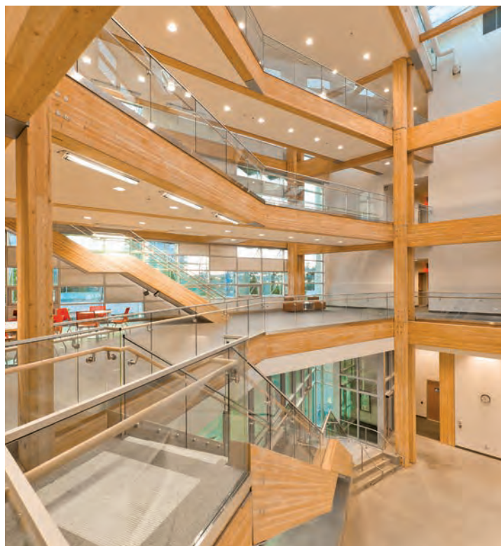
All of the wood for the CIRS building at UBC was from B.C., incorporating a variety of species and products including Douglas-fir glulam beams. Photo: Don Erhardt
