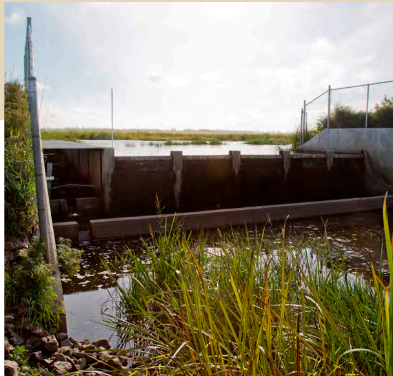
Water control structures regulate water flow in and out of wetlands helping to reducing flooding and drought./©Ducks Unlimited Canada
