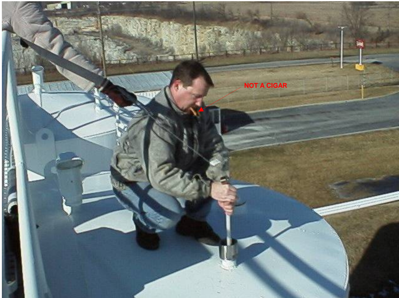
Figure 37 – Assembly of DataStik™-VB Fixed Bottom Probe
