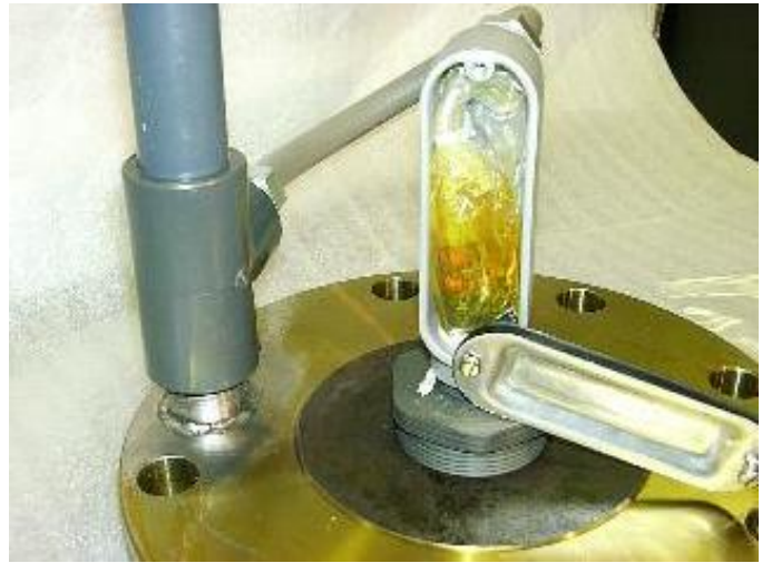
Figure 34 – Installing Wiring Into J-Box
