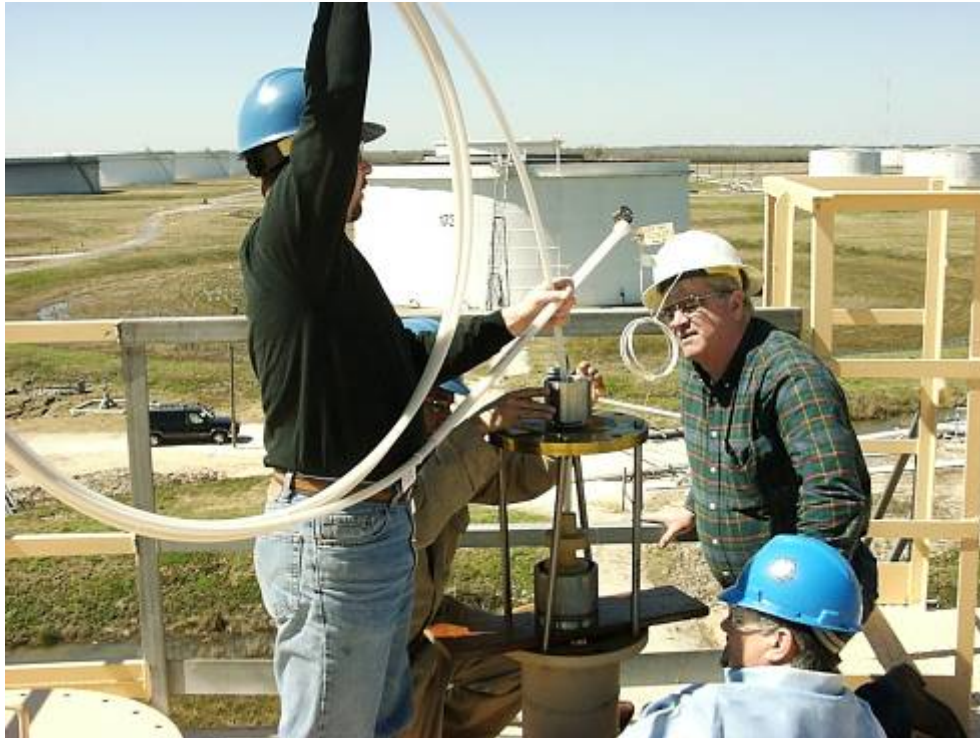
Figure 11 – Proper suspension of flange blind
