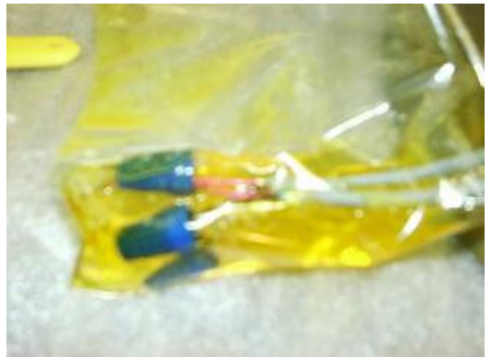
Figure 31 – Greasing the Wire Nuts
