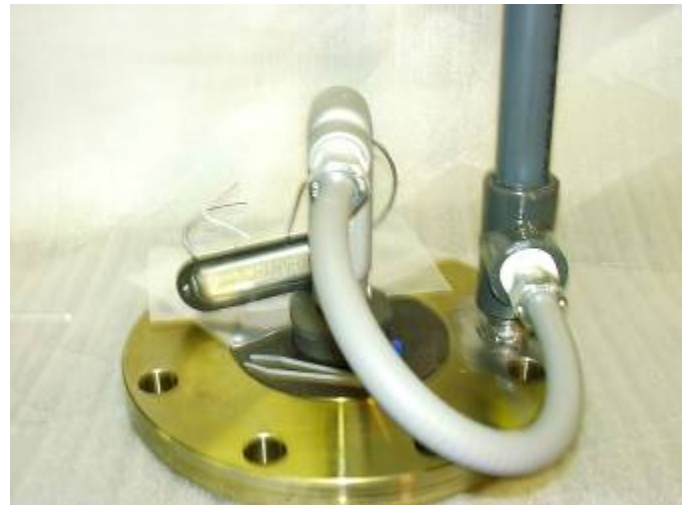
Figure 30 – Attaching Flexible Conduit
