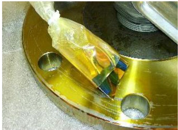
Figure 33 – Tie-wrapping Polybag
