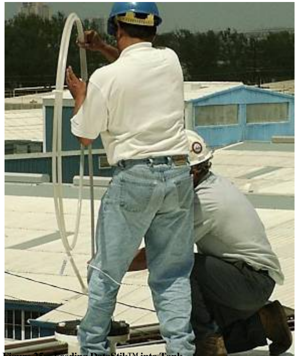
Figure 25 - Feeding DataStik™ into Tank
