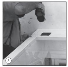
Brace the glass cap up to the header with the hinges facing up at the top. With the glass cap flush with the header edge, screw the hinge plate to the header with the black 1-1/2" screws.
