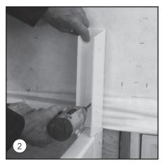
With the rear mounting plate centered over the well side and flush to the outside building wall secure with 2 Tapcons  $(3/16 \times 1-3/4)$  while ensuring that the plate remains plumb.
