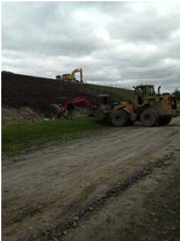
Fig. 3 Mini excavator for ditch cleaning cell 3 and cell 4
