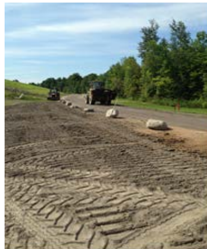
Fig. 2 Landfill Road Maintenance
