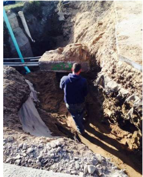
Fig. 4 – Backfilling sewer lines from the new maintenance building on November 11, 2015.
