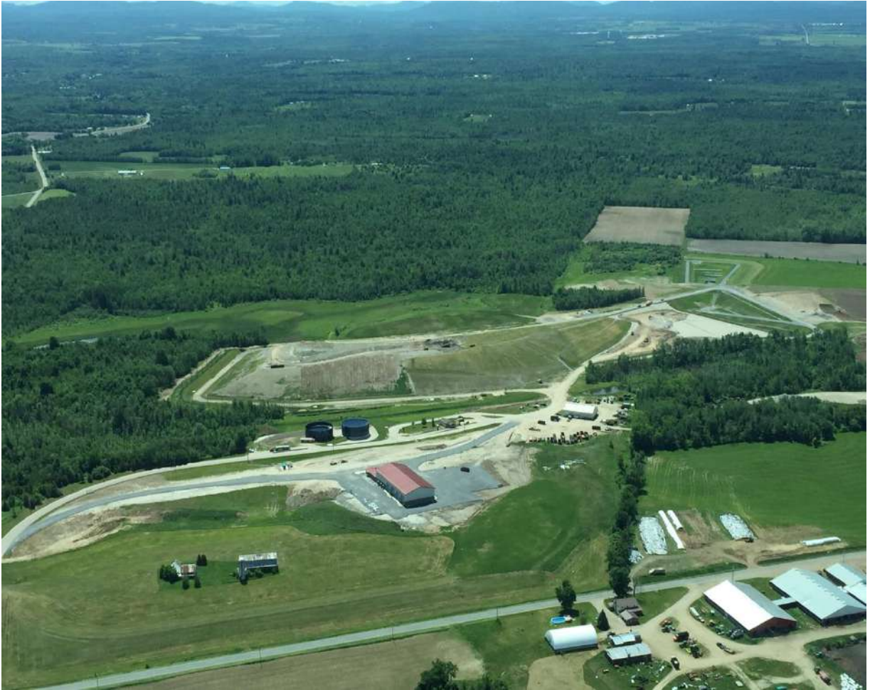
CFSWMA FRANKLIN COUNTY LANDFILL SITE
