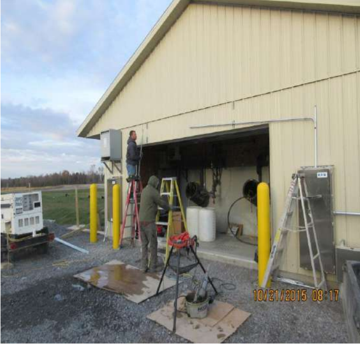
Fig. 6 – Watson Electrical working on the Side Riser Building on October 21, 2015.
