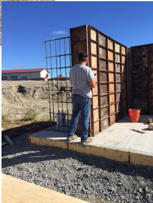
Fig. 8 –Placing forms for concrete pour on convenience station
