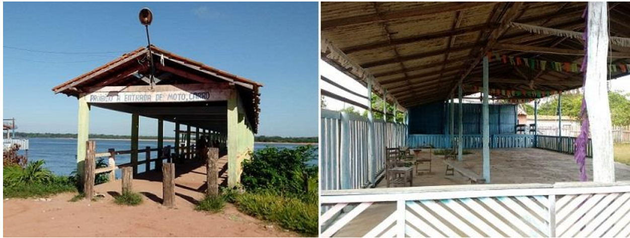
Figure 3 - Dock in Vila Ituquara (left) and Community Center in Vila Matacurá (right).
