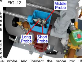
probe. Remove probe and inspect the probe rod. If sediment has accumulated, use a stiff wire brush to remove it. Install the probe in its place in the column and connect the wire back to the probe.
