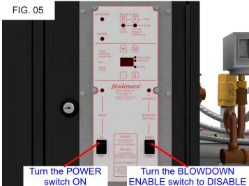
After approximately 2 seconds, the WATER FEED light turns on and water enters the boiler. As soon as the water level reaches approximately half height in the gauge glass, the automatic water feed turns off.
