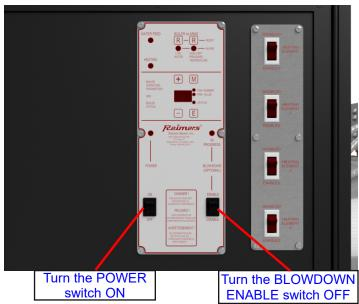
f. After approximately 2 seconds, the WATER FEED light turns on and water enters the boiler. As soon as the water level reaches approximately half height in the gauge glass, the automatic water feed turns off.
