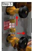
Slide glass up, pull out on bottom of glass and remove
