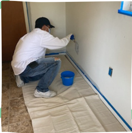
A Hope Works client works to paint and prepare Hope Commons
