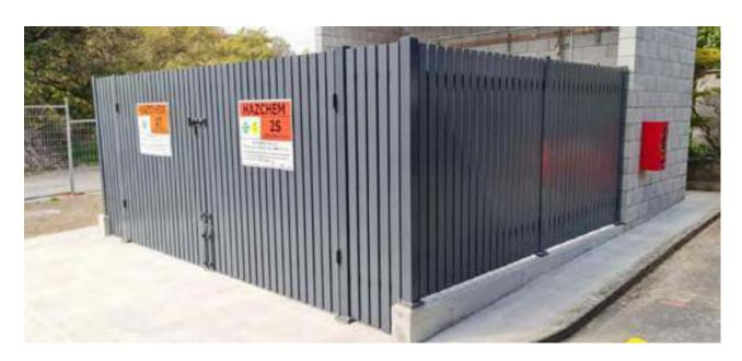
Commercial gas bottle storage area. – Grey Friars vertical face fixed slat option. 2000mm high with Flanged fixed 90x90mm posts.
