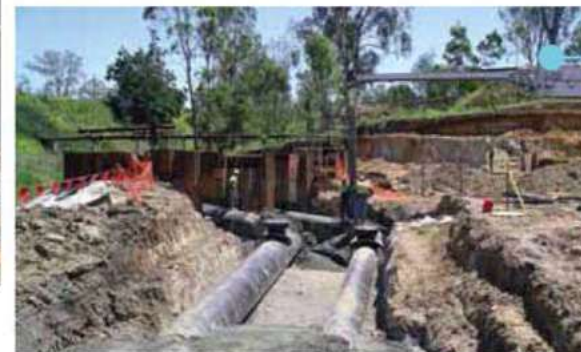
Placing stabilised sand around pipes, where safe direct access by wheel loader or excavator is impossible. All material can be placed from the side most accessible to vehicles.
