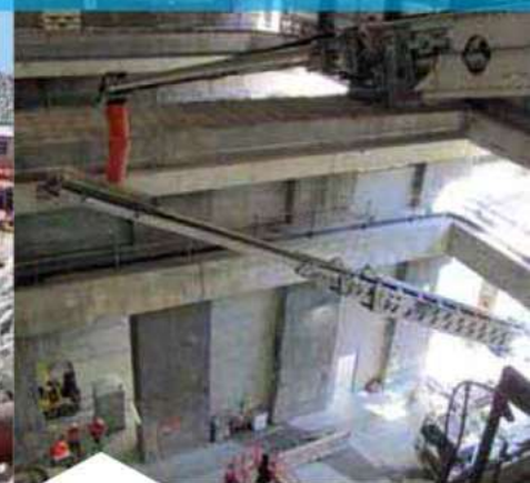
passing concrete from the surface for paving a tunnel floor
