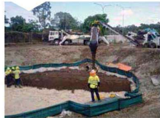
Backfilling over geotextile in a detention basin
