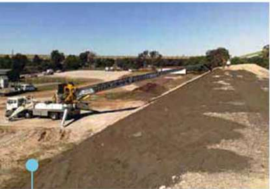
Placing soil on a noise wall: a productive alternative to other methods in areas that cannot be accessed directly or safely. Mulch and bark can also be placed, and belt speed and discharge height can be adjusted to suit cellular confinement systems.
