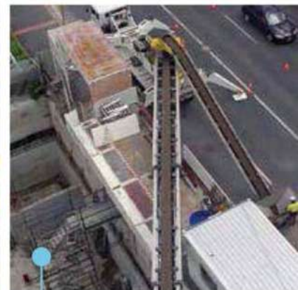
Going down ... placing crusher dust in a basement.
