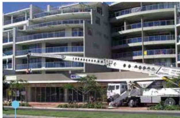
Going up ... placing drainage gravel for a mezzanine level garden.
