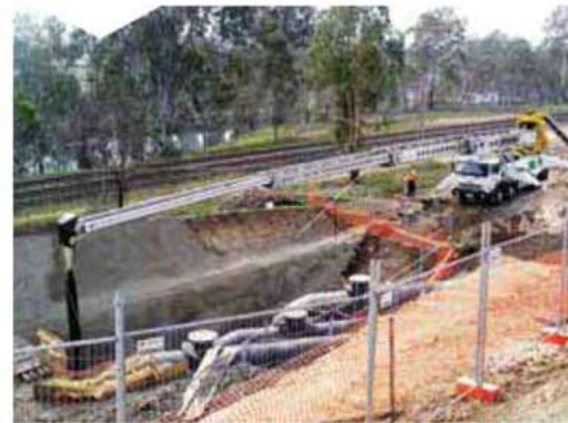
Placing unpumpable concrete
