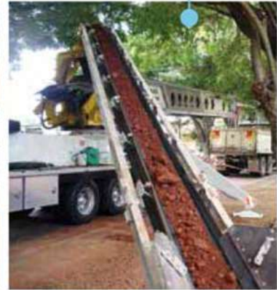
Removing soil from a basement excavation and direct loading a tipper on the street. This avoids the tipper entering the site, and often the need for a wheel wash at the site exit.
