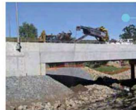
Placing stabilised sand around pipes, where safe direct access by wheel loader or excavator is impossible. All material can be placed from the side most accessible to vehicles.
