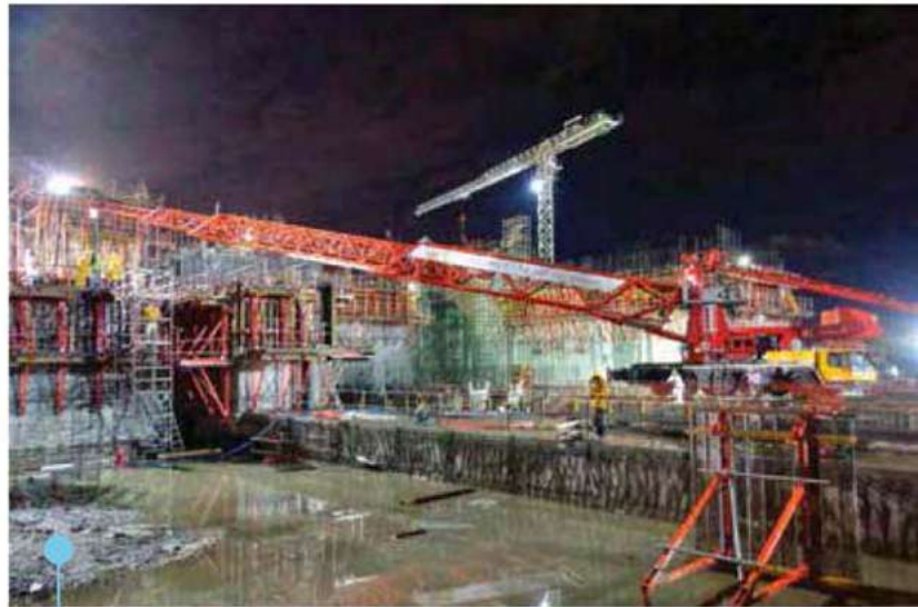
With 61 metres of reach, the TB 200 covers a huge area for mass concrete pours, without the need to relocate.
