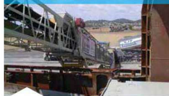
Radial stacking conveyors
