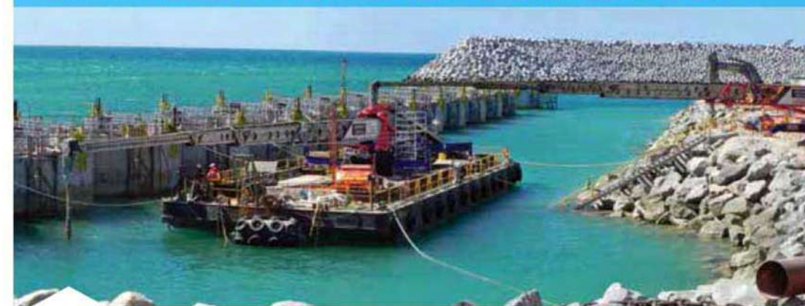
passing concrete from shore via a barge for an underwater pour
