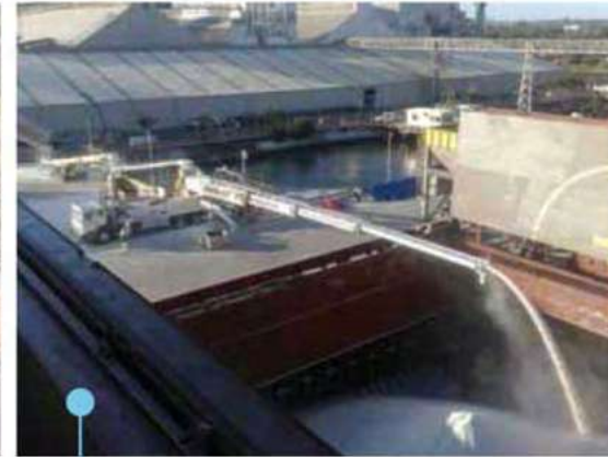
Loading urea into the hold of a ship at a general purpose wharf. The telescopic slewing discharge belt facilitates even placement of the bulk cargo in the hold.
