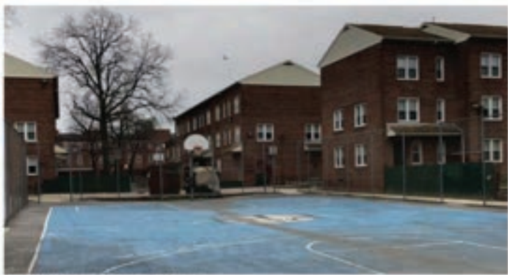
BASKETBALL COURT (PRIOR TO RESURFACING)
