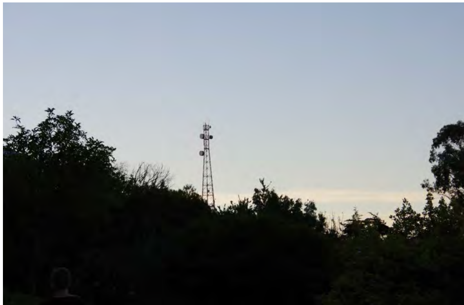
Low population density creates little market incentive for providing internet and cellular services in rural areas. Filling broadband and cellular service gaps is critical for economic growth.
