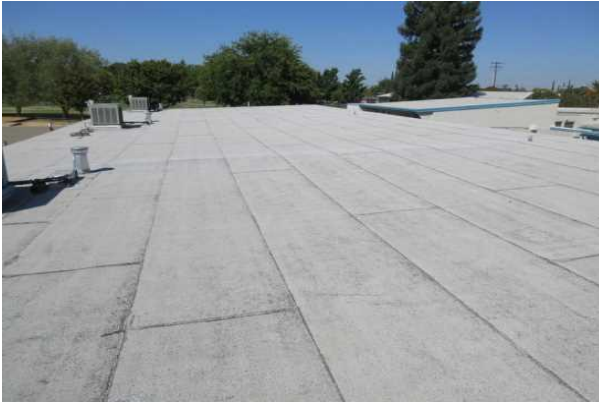
#19 MODIFIED BITUMENOUS ROOFING
