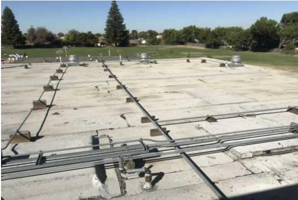
#15 TYPICAL MODIFIED BITUMEN ROOFING
