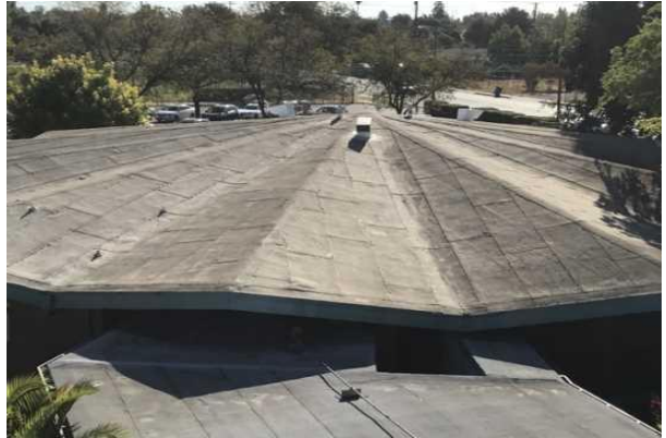
#16 FOLDED ROOF MODIFIED BITUMEN
