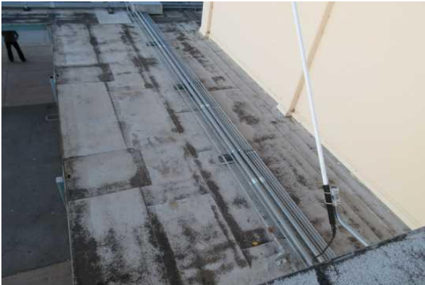
#17 COVERED WALKWAY ROOFING
