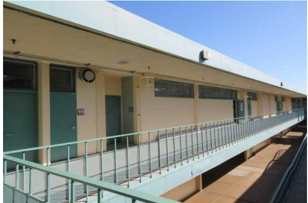
#20 SECOND FLOOR WALKWAY
