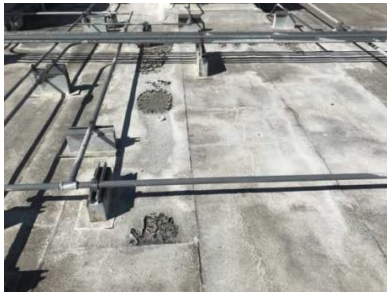
Roof is bubbled and peeling. - AssetCALC ID: 1475960
