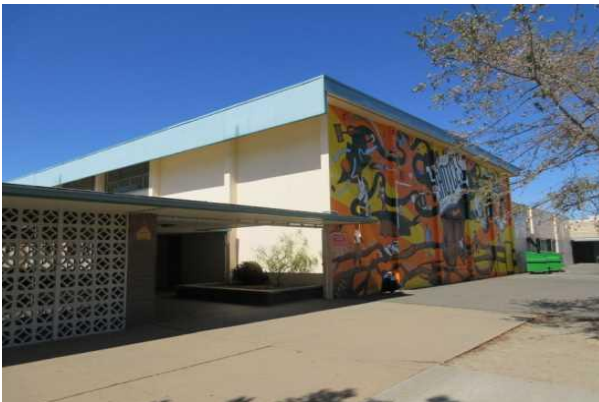
#5 FRONT ELEVATION-BLDG 00F, MPR
