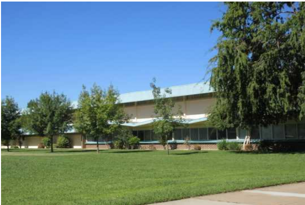
#3 FRONT ELEVATION-BLDG 00A AND 00B
