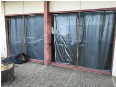
Doors are single pane glazed, energy inefficient and well past EUL. Their size makes them very difficult to operate. - AssetCALC ID: 1475729
