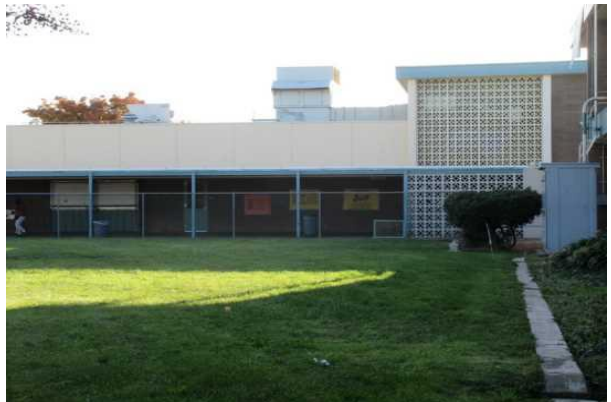
#6 REAR ELEVATION-BLDG 00F, MPR
