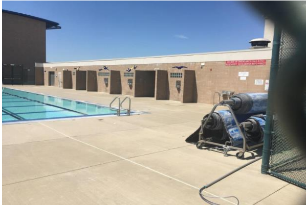
#9 POOL BUILDING (H)
