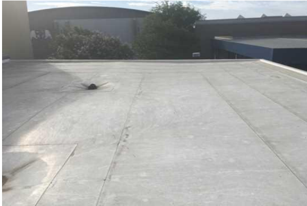
#13 ROOF, SINGLE-PLY TPO/PVC MEMBRANE
