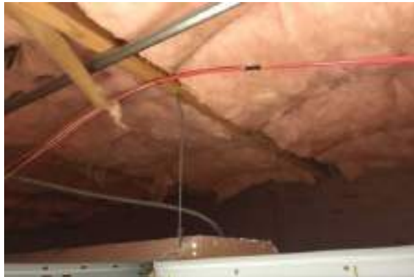
#21 ATTIC SPACE PORTABLE 21
