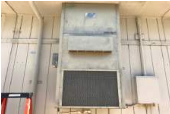
#29 WALL-MOUNTED HEAT PUMP
