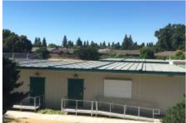
#14 METAL ROOF, PORTABLES
