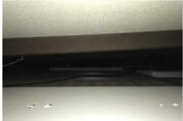
#20 ATTIC SPACE PORTABLE 18
