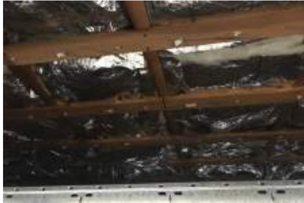
#19 MAIN BUILDING ATTIC SPACE
