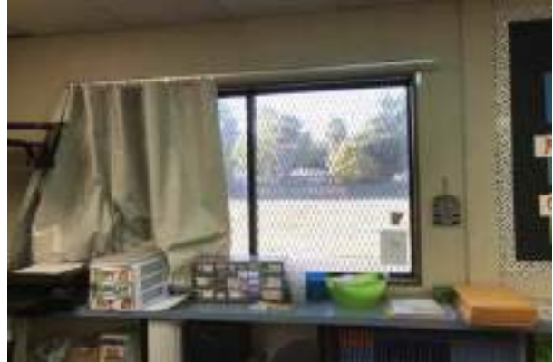
#20 PORTABLE BUILDING WINDOW
