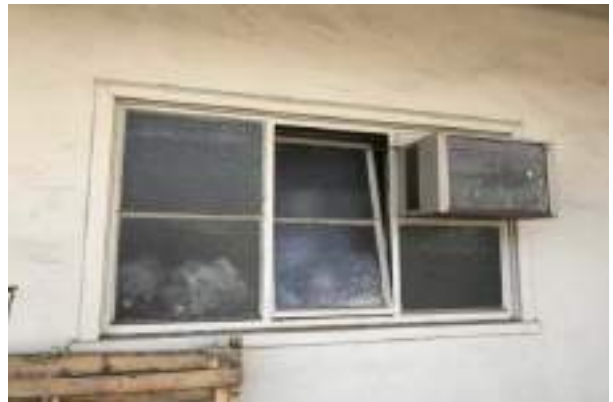
#18 ORIGINAL WINDOWS, BUILDING 1
