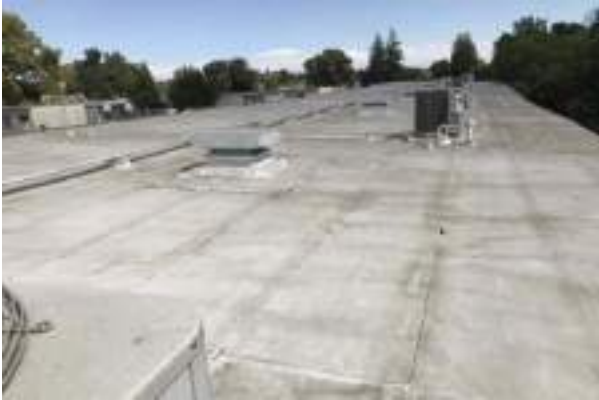
#13 ROOF, BUILDING P02
