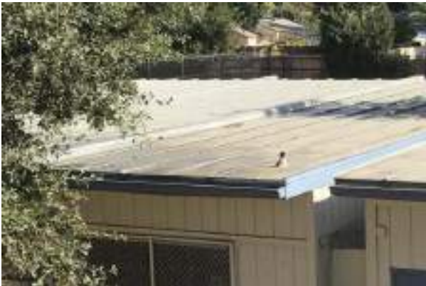
#15 METAL ROOFS AT PORTABLES
