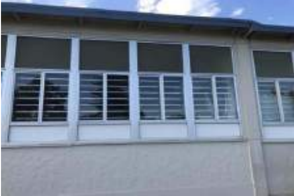
#19 REPLACEMENT WINDOWS, BUILDING P02
