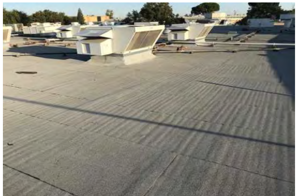
#42 MODIFIED BITUMEN ROOF
