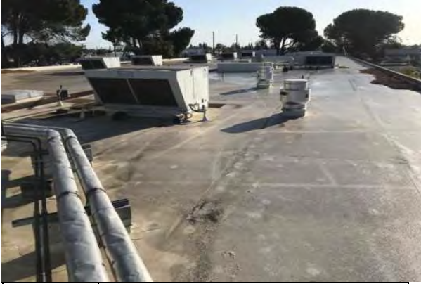
#43 SINGLE-PLY TPO ROOF
