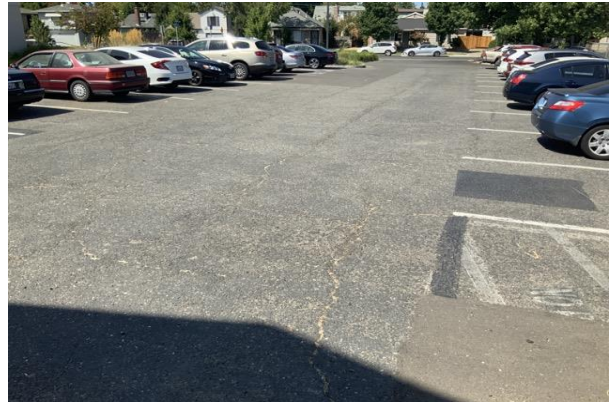
#6 ASPHALT PARKING LOT
