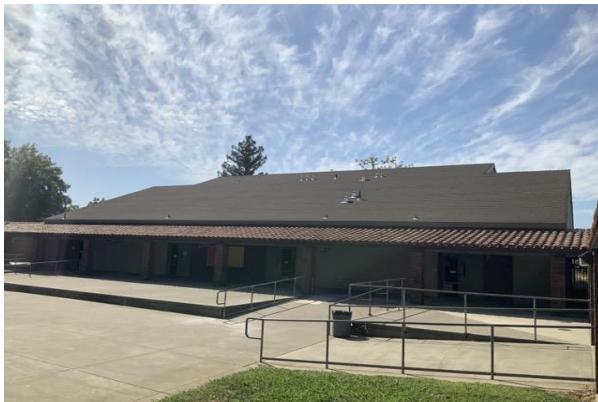
#11 ROOF, ASPHALT SHINGLE
