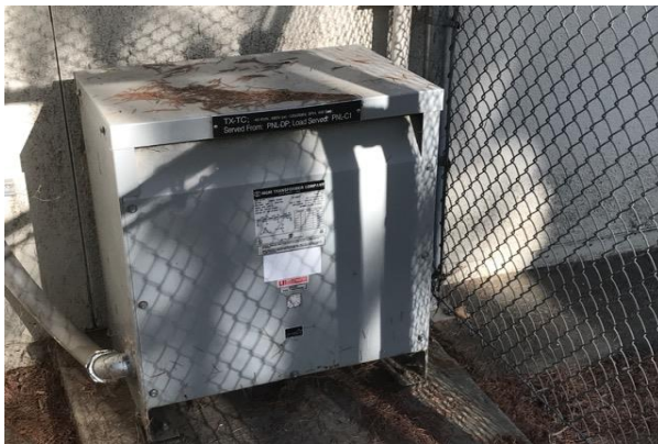
#21 SECONDARY TRANSFORMER, DRY, 45 KVA, REPLACE
