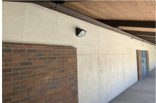
#14 EXTERIOR STUCCO AND BRICK
