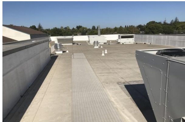
#12 ROOF, SINGLE-PLY TPO/PVC MEMBRANE
