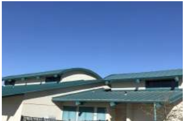
#24 ROOF BUILDING K
