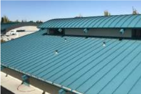
#25 ROOF BUILDING C
