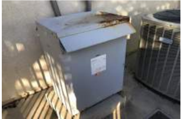
#38 SECONDARY TRANSFORMER
