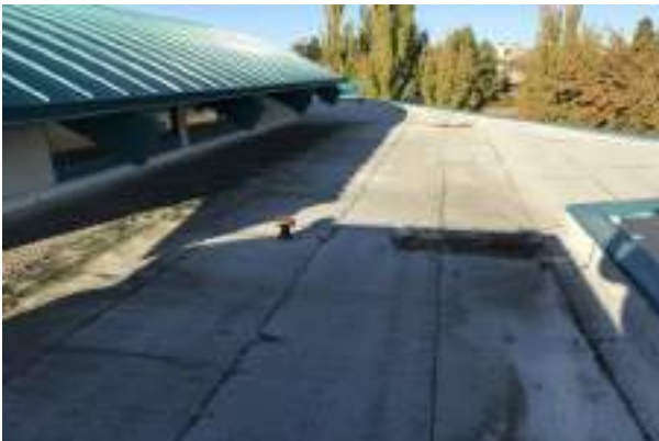
#23 ROOF ADMINISTRATION BUILDING
